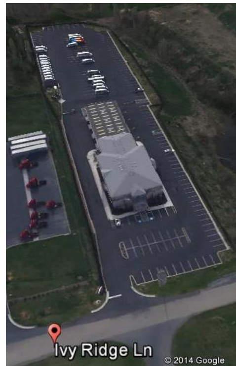
Overview of Facility
